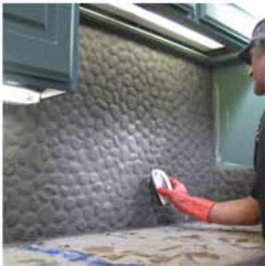
Sweep out more grout with a brush
