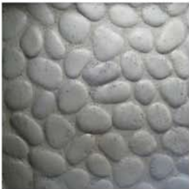
Grout is recessed
